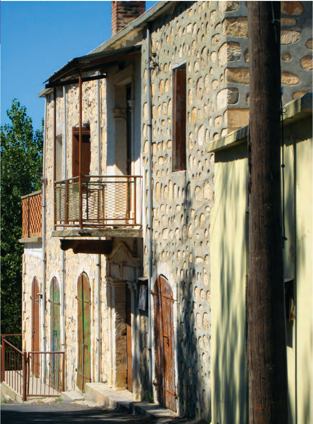
▲ Stonebuilt houses in Drouseia.
